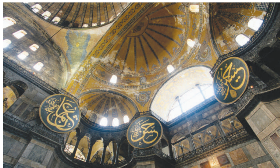
Ancient innovation: triangular ‘pendentives’ join supporting arches to the building’s enormous dome.
